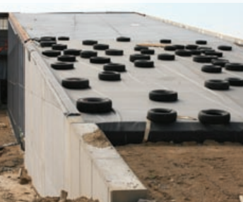
1 Install slipsheet/root barrier
