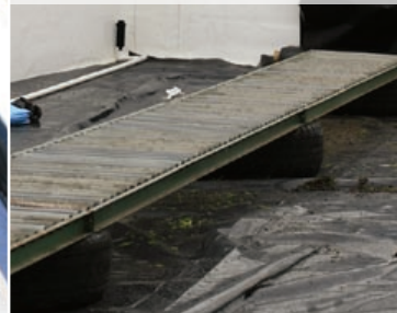
3 conveyors set up
