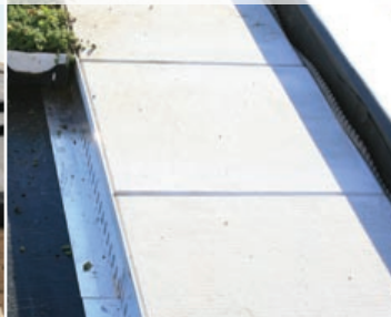
2 Install edging and pavers
