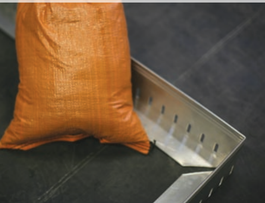
9 edging held in place with temporary ballast
